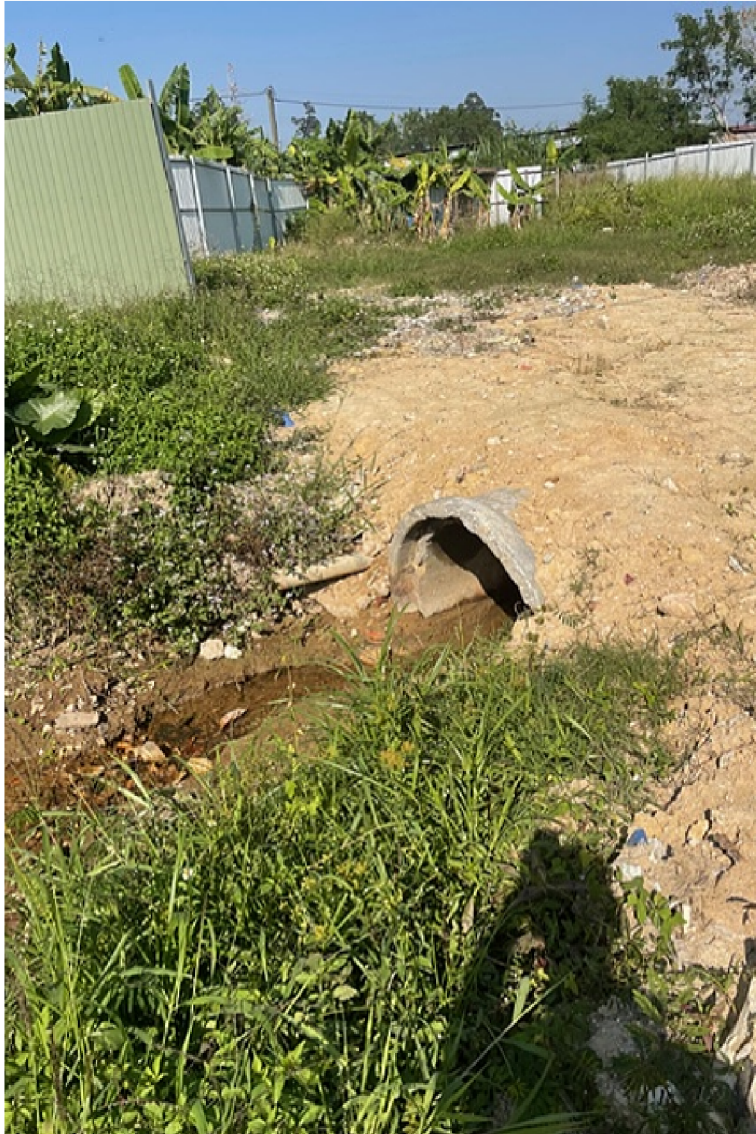
Photo 2 - 1m dia. pipe
